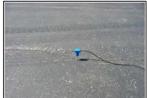
Figure 5. View of typical geophone secured into pavement prior to surveying.
